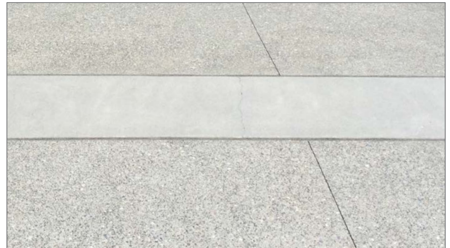
Example of acid-etched cement concrete pavement with smooth bands
