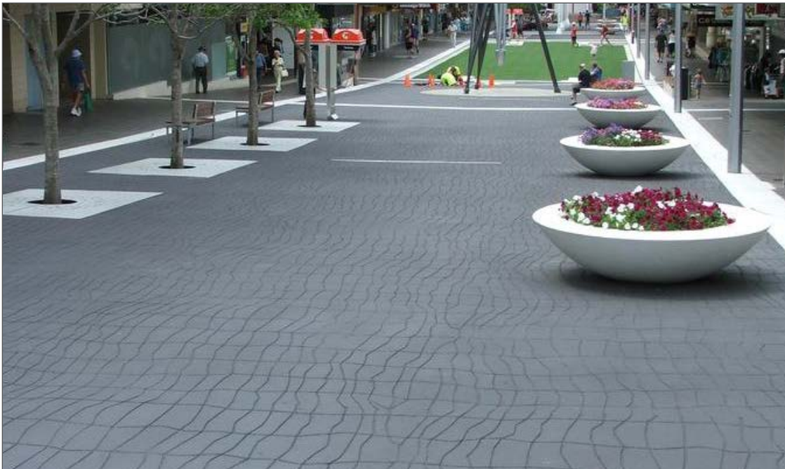
Example of stamped colored cement concrete pavement
