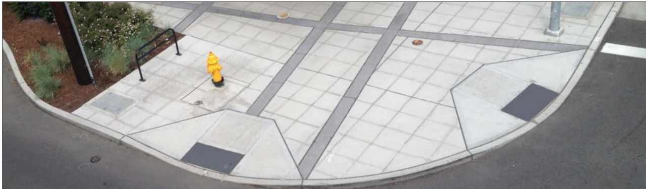
Example of accent pavement with 2' x 2' angled grid scoring and linear accent bands
