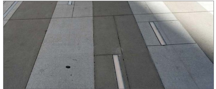
Example of scored colored cement concrete pavement
