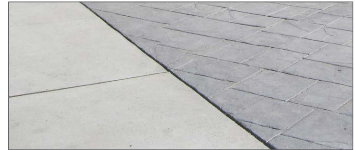
Example of contrasting smooth and stamped cement concrete pavement
