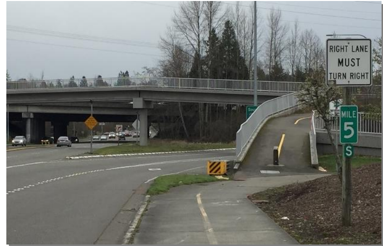
44th Ave W Pedestrian Bridge/Interurban Connection
