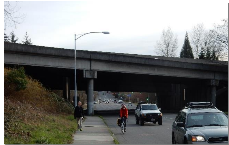
I-5 and 44th Ave W Interchange
