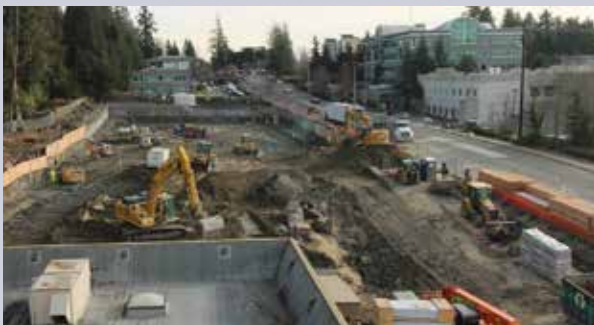
Community Justice Center construction
