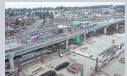
Construction continues at the Lynnwood City Center Station
