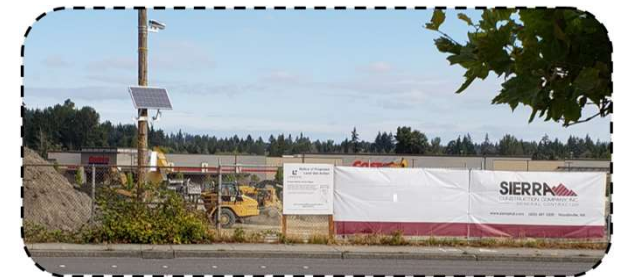
Future site of Home Depot
