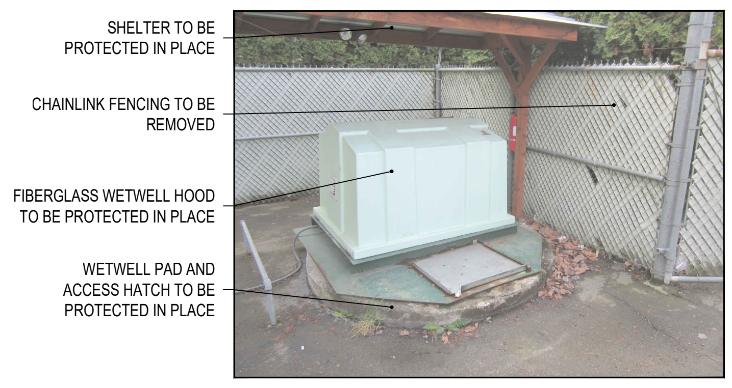
EXISTING SITE PHOTO
