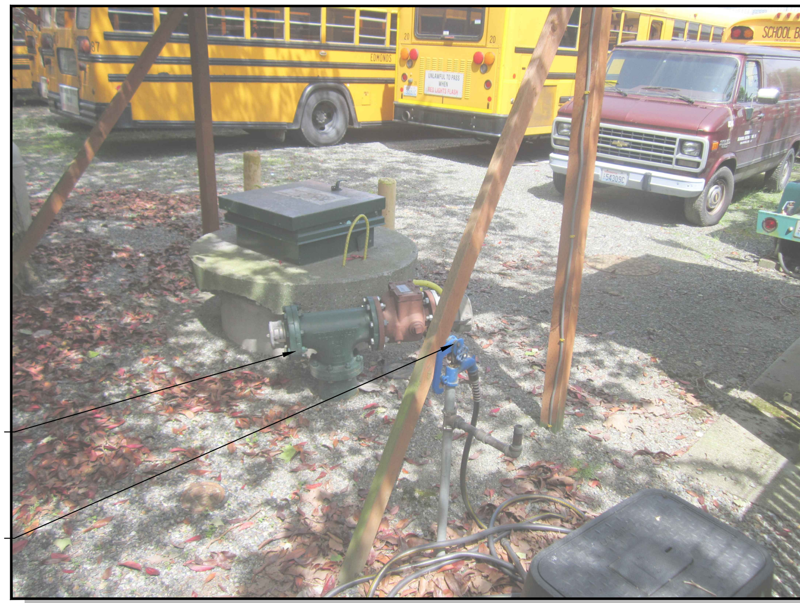
EXISTING SITE PHOTO
