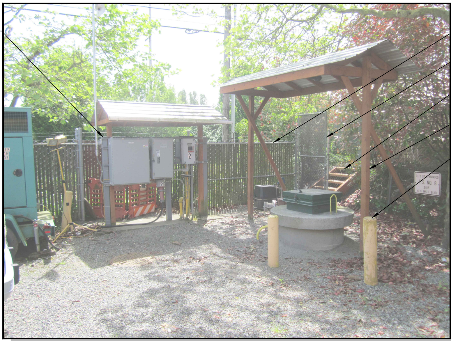
EXISTING SITE PHOTO
