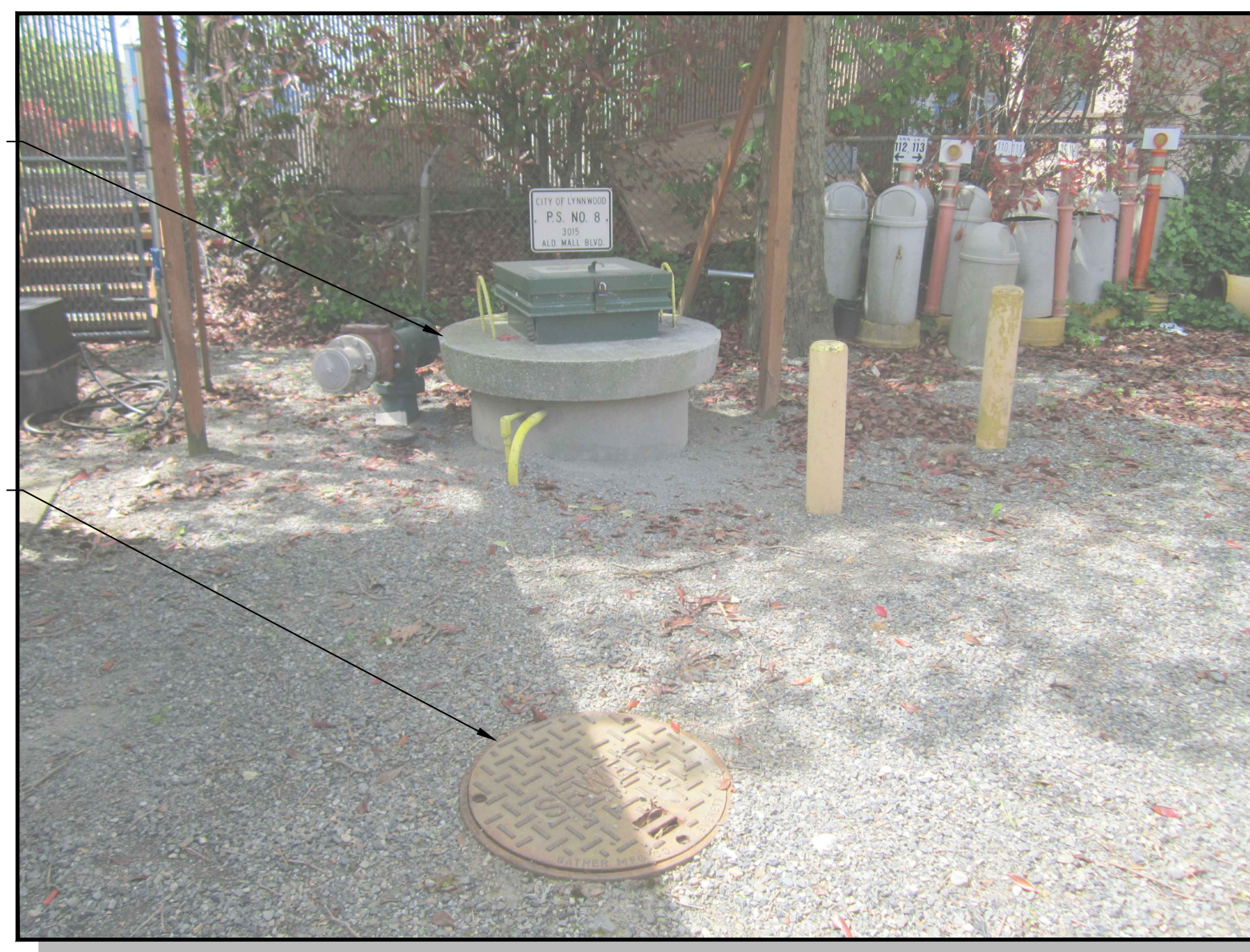
EXISTING SITE PHOTO
