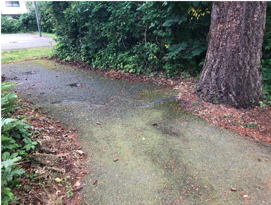
4 5 6 7 Figure 4 - Asphalt in the critical root zone (CRZ) will be demolished. A large root from tree #1128 travels only a few inches below the surfacing where the asphalt has heaved. These areas should be hand-worked to avoid damaging the roots. (photo on July 2, 2018)
