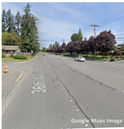
36th Ave West at 192nd PCI = 74 Chip Seal Candidate
