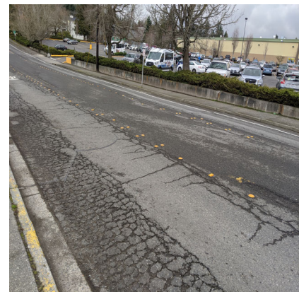
48th Ave West north of 196th PCI = 33 Full-Depth Reconstruction 2021 program
