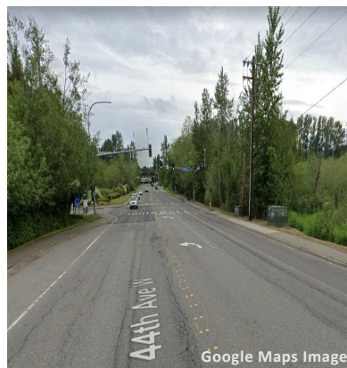
44th Ave West at 20800 Block PCI = 54 Grind/Overlay 2021 program
