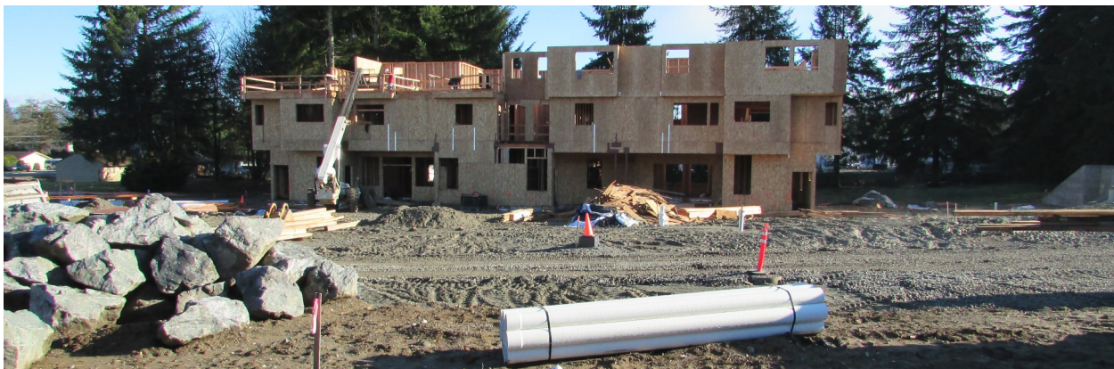
Housing Hope's Monroe Family Village under construction.
