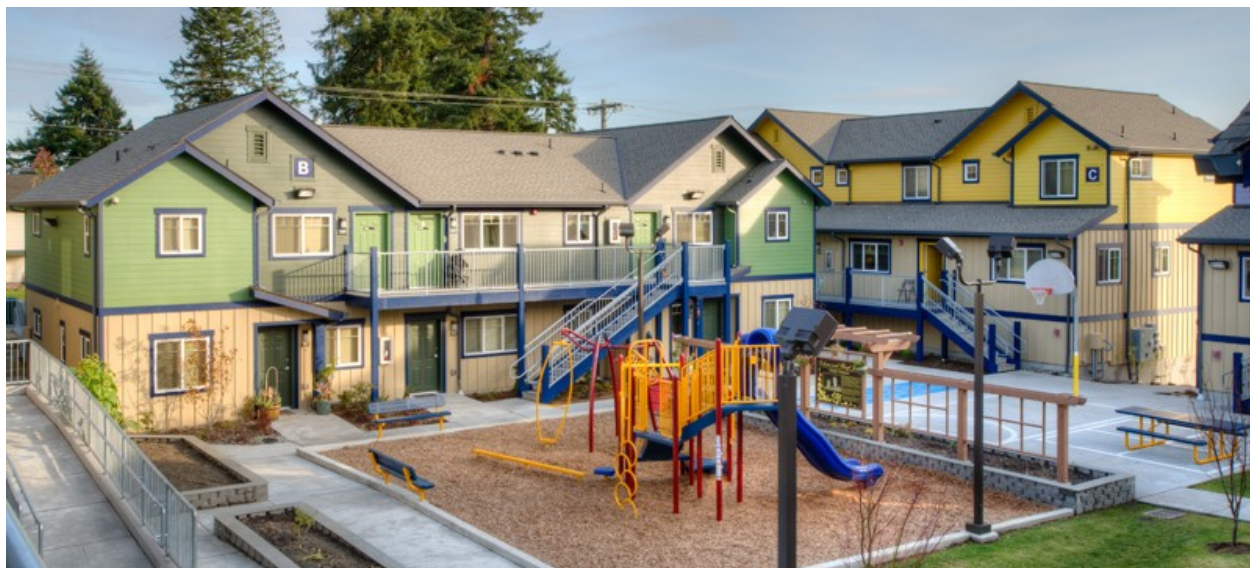
Housing Hope's Lincoln Hill Apartments, in Stanwood.
