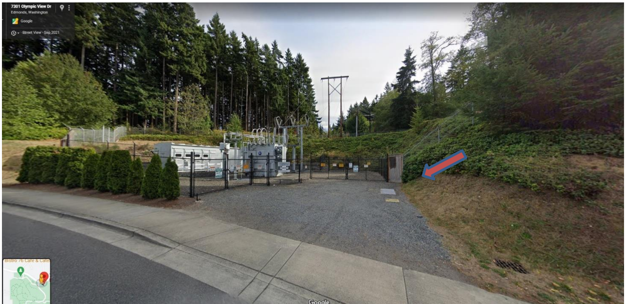
Figure 2. Project location, Google Street view image from Olympic View Drive (taken September 2021), view facing towards the project site. Arrow depicts location of proposed AMI pole.
