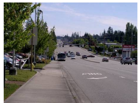
Figure 3. Highway 99 features a 7-lane section with sidewalks.
