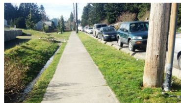
At-grade concrete walkway with wheel stop delineators
