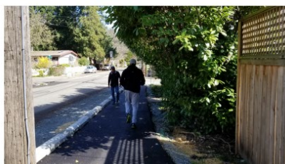
At-grade asphalt walkway
