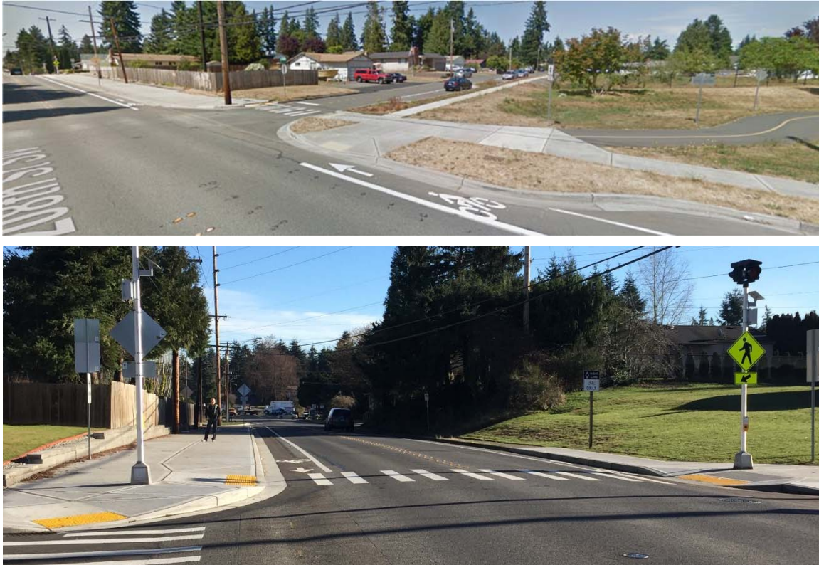
Figure 22 Interurban Trail Sidepath and Crossing at 208 th Street SW, Lynnwood, WA
