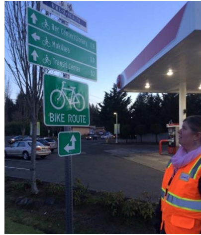
Bicycle route signage is placed low to the ground and obstructs travel along the sidewalk.
