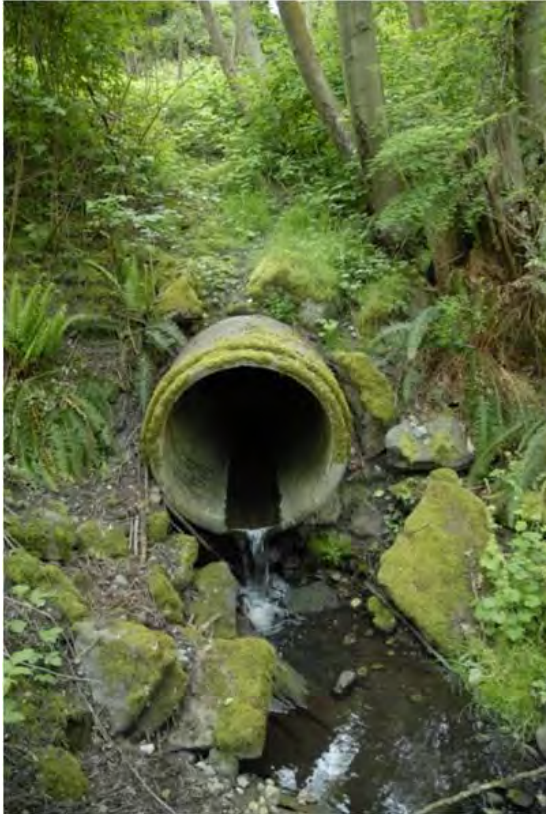
Photo 4-32. Clear groundwater seepage.
