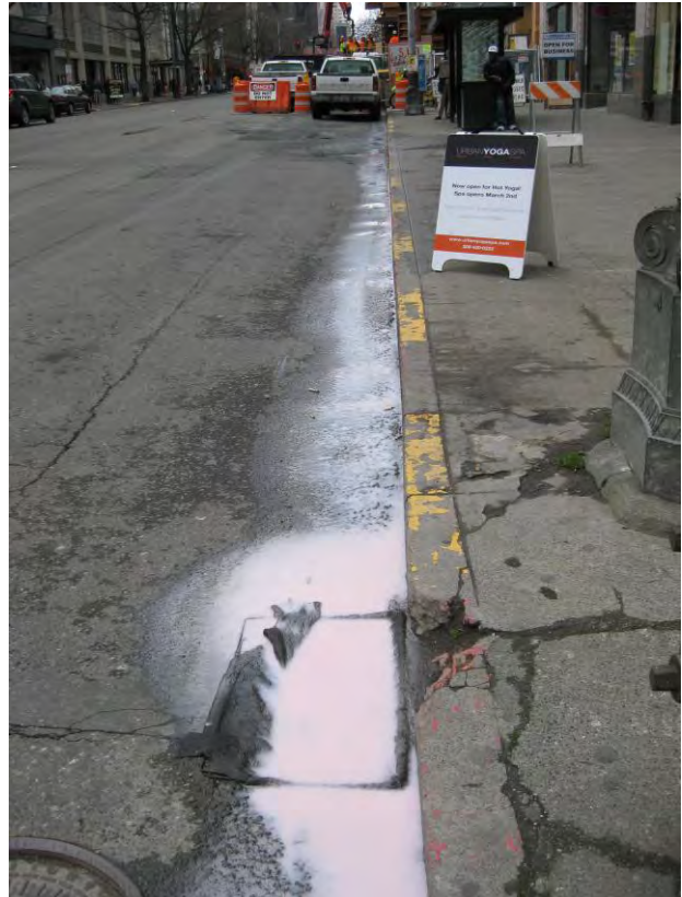
Photo 4-25. Drywall mud discharge.
