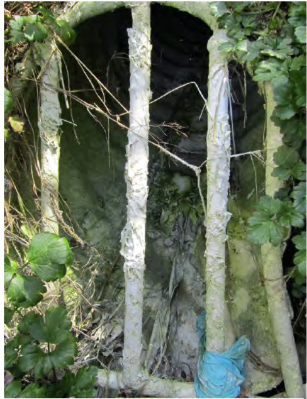
Photo 4-9. Paint from commercial painting company.
