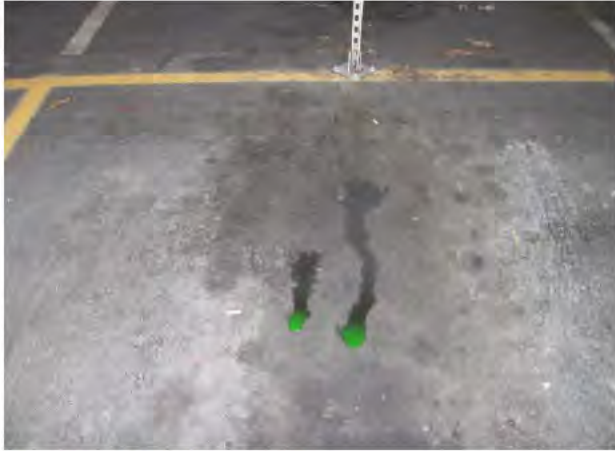
Photo 4-12. Antifreeze spill.
