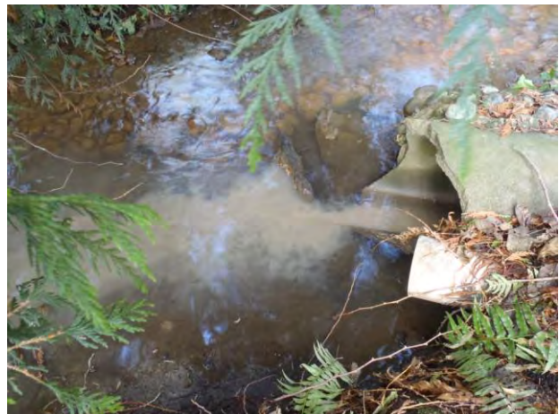
Photo 4-27. Turbid discharge.
