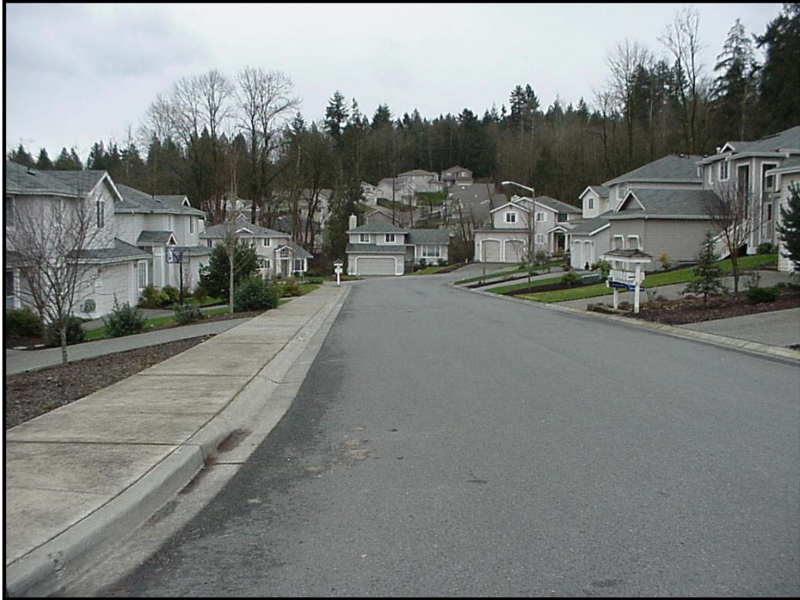
Figure 7. Urban stormwater. If there was such a thing as a pollution smorgasbord, urban stormwater would be the ultimate dining experience. Laden with fertilizer, pesticides, petroleum products, heavy metals from tire wear, storm sewers rapidly convey these pollutants from the road above to local streams in most of western Washington whenever it rains.
