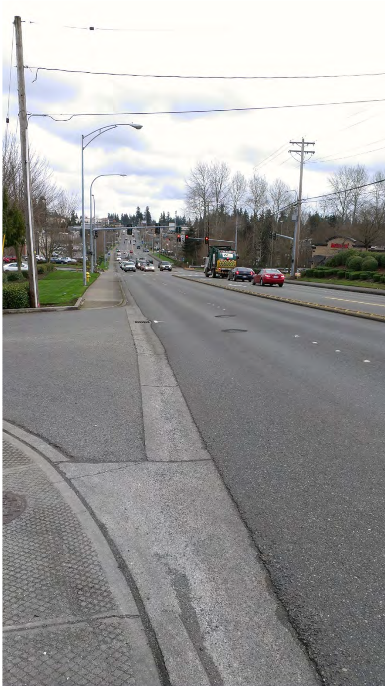
Photo 400: Beginning of TDA 2 downstream route. 196th Street SW facing east.
