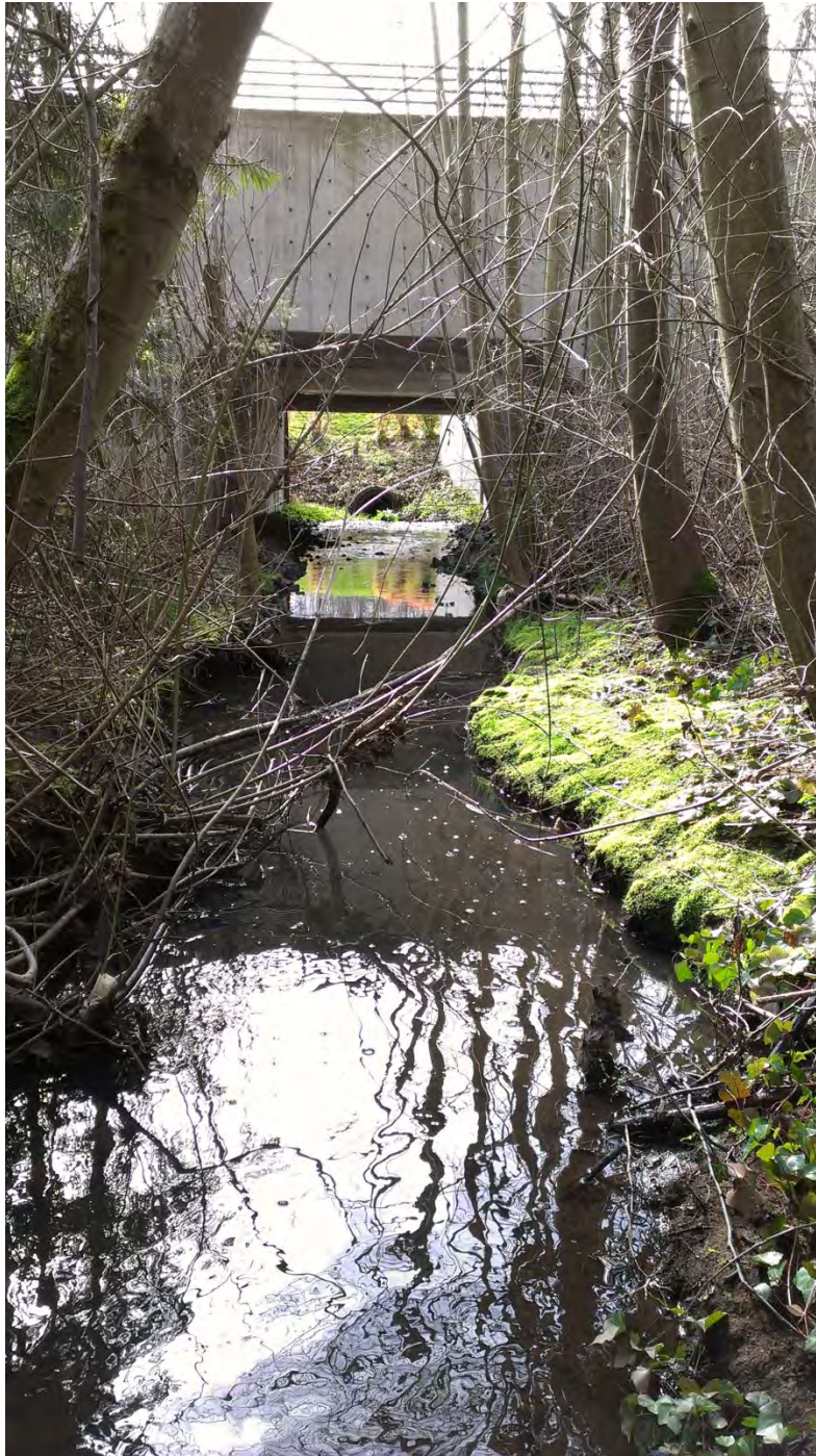
Photo 109: Golde Creek facing south, approximately 300 feet north of 196th Street SW.
