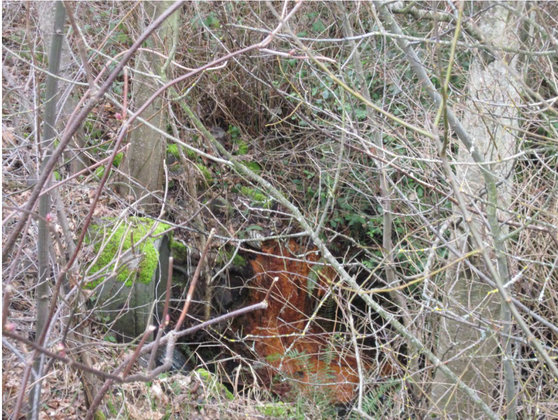
Photo 404: Golde Creek outfall on the south side of 196th Street SW. Photo facing east, creek flowing south.
