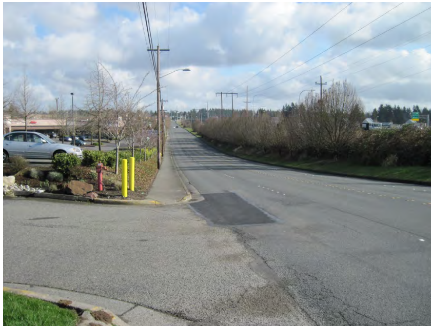
Photo 100: Start of TDA 1 Downstream Route. Alderwood Mall Boulevard facing northeast.
