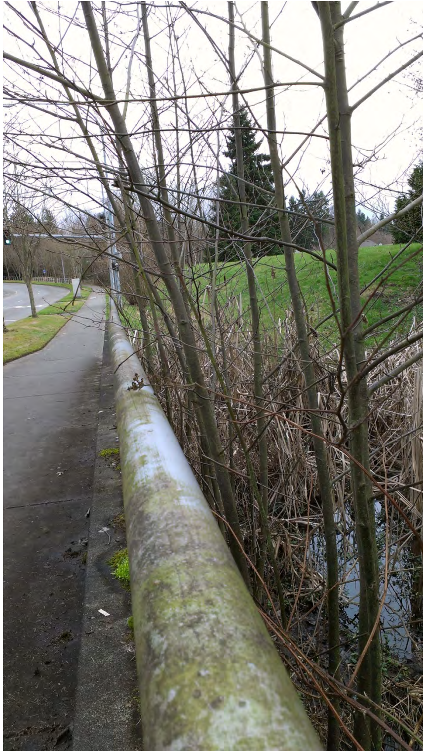
Photo 605: Downstream of pond, Alderwood Mall Parkway facing east.
