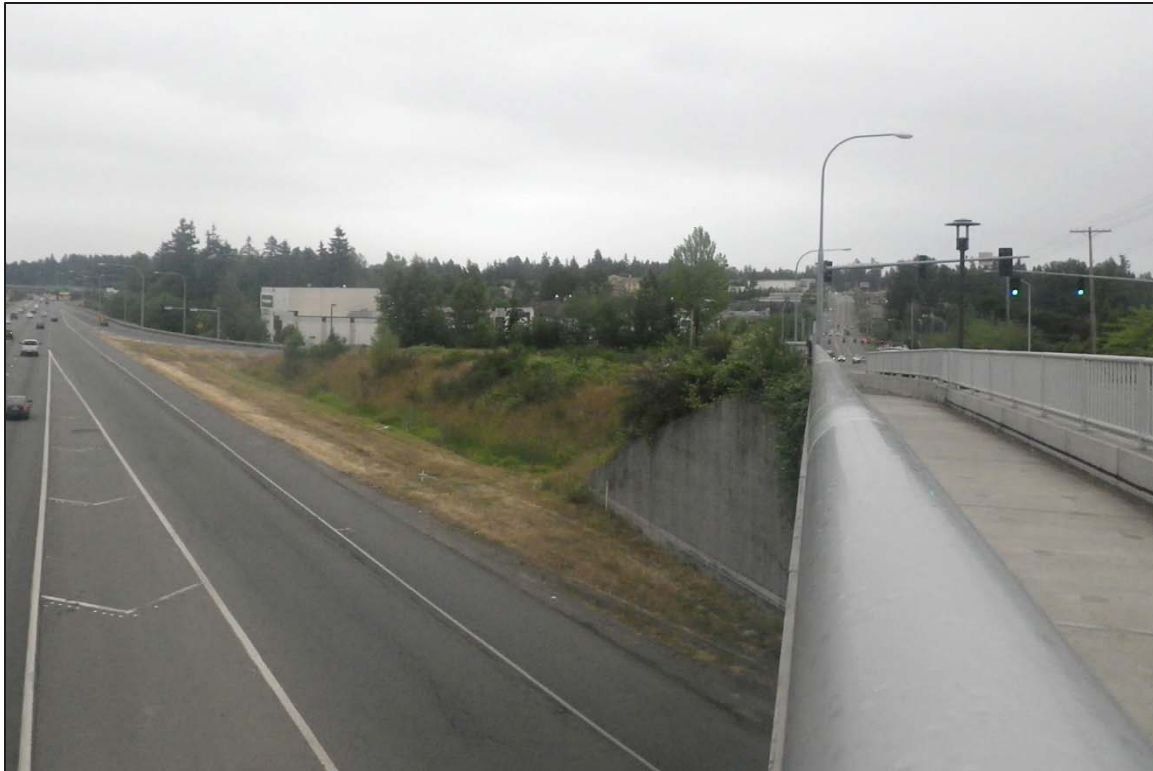
Figure 10. Overview of the modern Interurban Trail from the overpass on 196 th St SW, view to the northeast.
