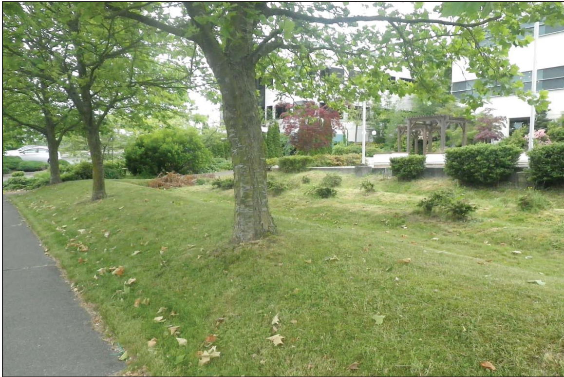
Figure 6. Overview of cut slope and land modification on the west side of 33 rd Ave W, view to the west-southwest.
