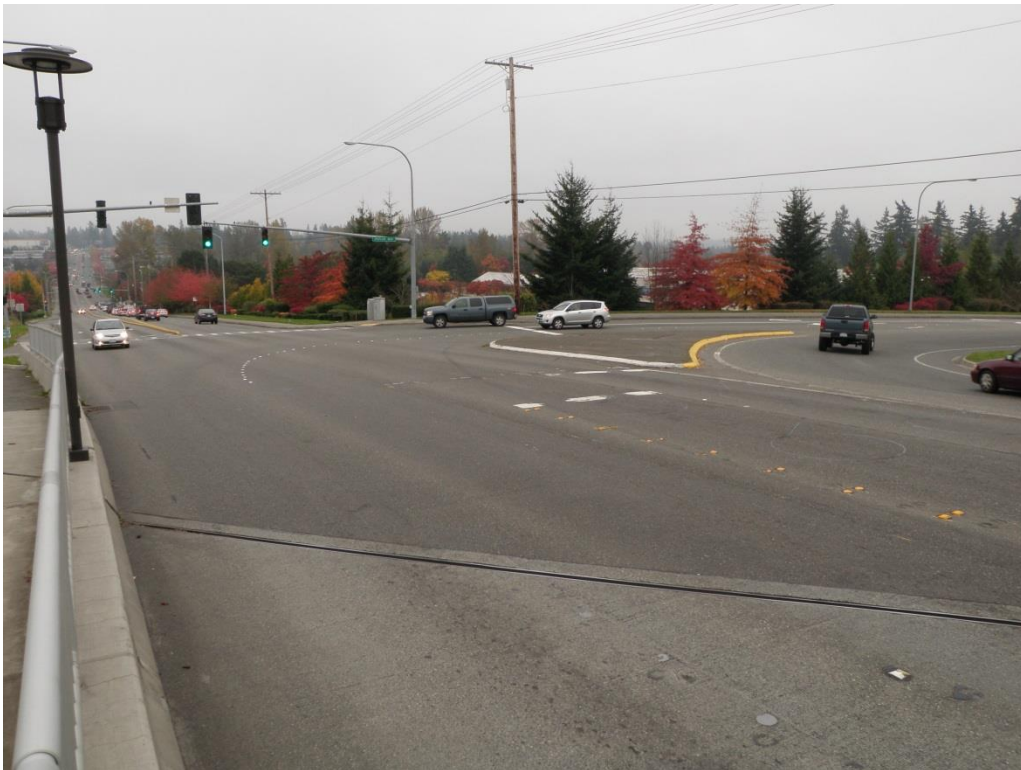
Photo 2—Intersection of 196 th Street SW and Poplar Way looking east
