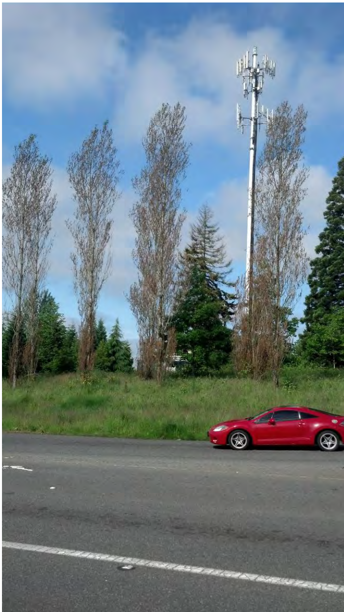
Cellular tower adj SW of Poplar Way/196 th Street SW intersection
