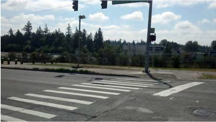
Poplar Way/Alderwood Mall Blvd intersection, view south
