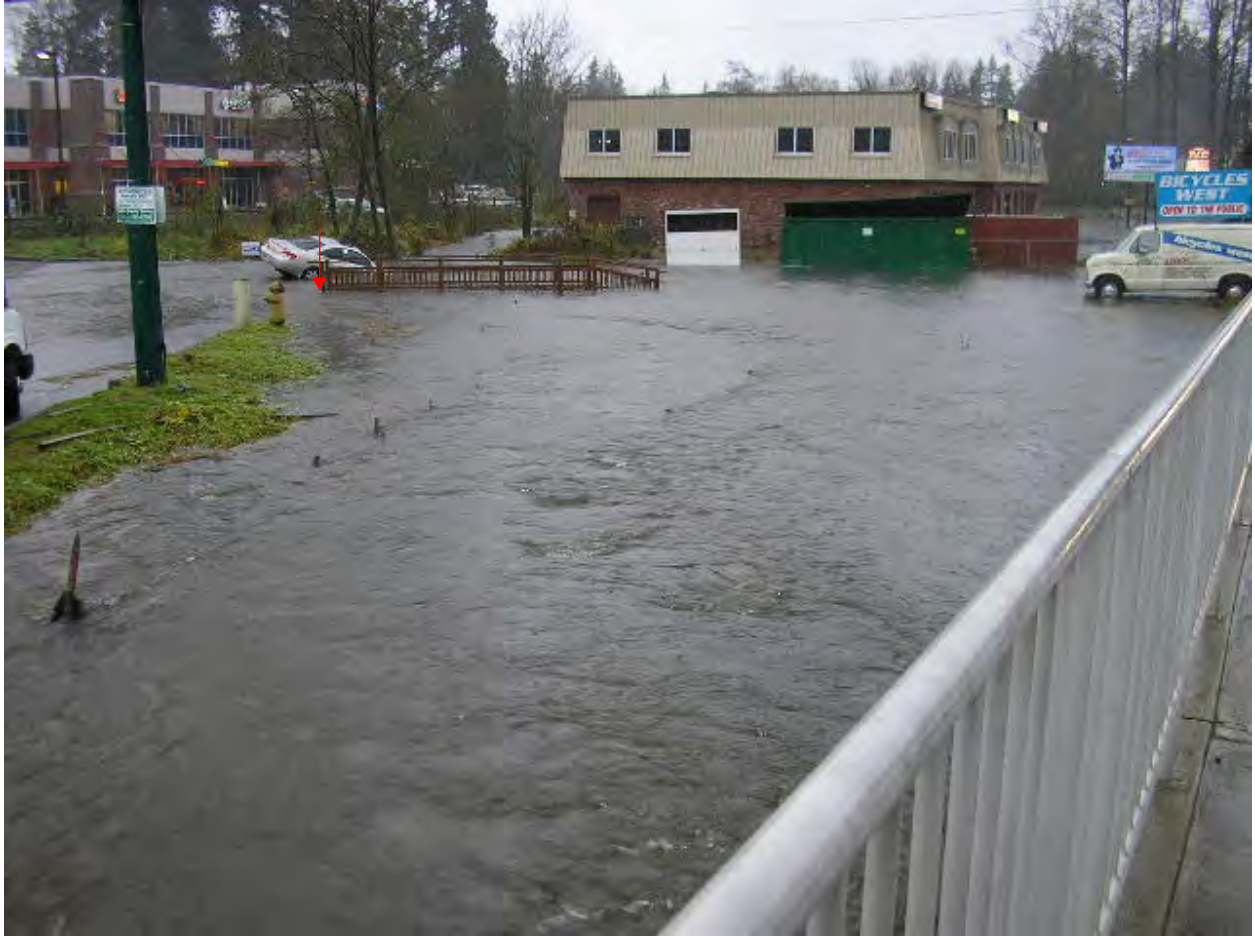
Photo 5: Bridge at Flynn's Carpet. December 2007
