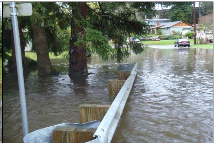
November 19, 2012 flooding of 190th St SW, looking west.
