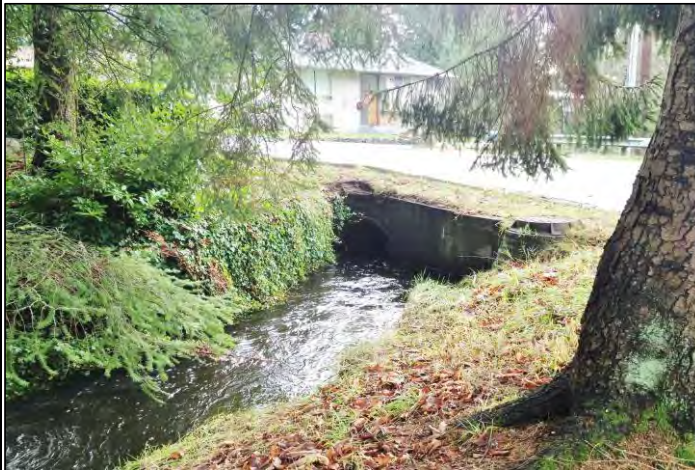
Looking downstream to inlet of existing 189th St SW culvert.
