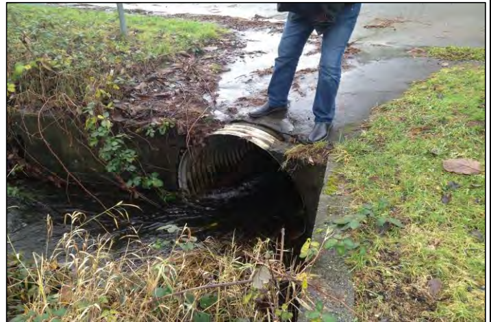
Looking downstream to existing culvert inlet at 191st ST SW.
