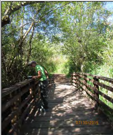
Existing Trail bridge crossing downstream of Scriber Lake.
