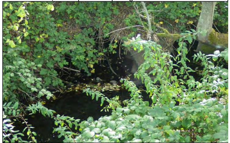
Looking down to inlet of existing 196th St SW culverts.
