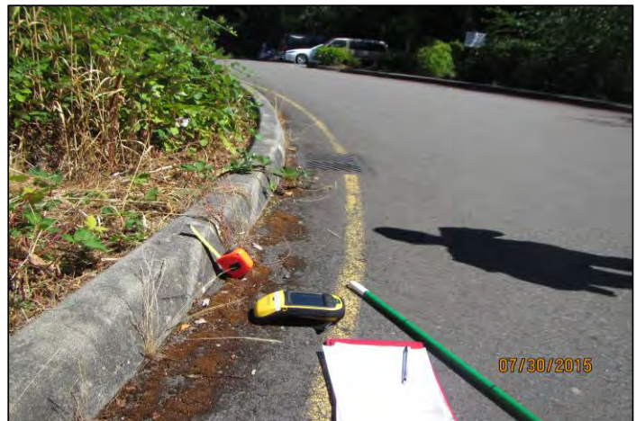
Curb within Eunia Plaza parking lot that berm could tie in to.
