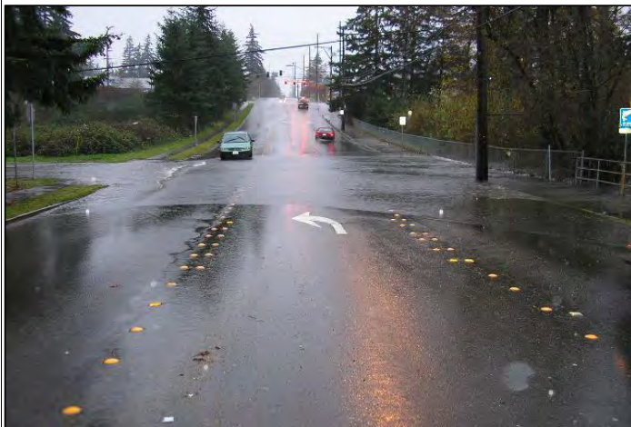
December 4, 2007 overtopping of 188th Street SW.
