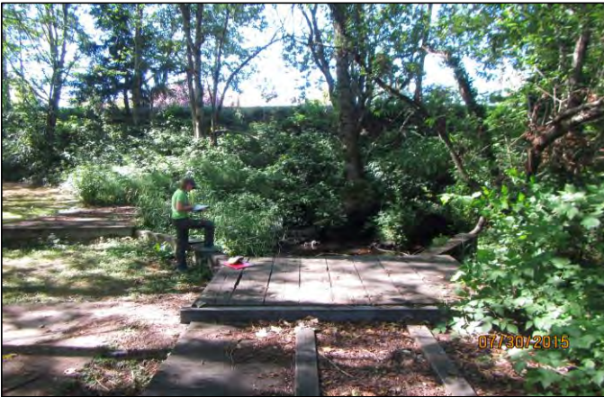
Looking upstream to diversion weir and vault during summer baseflows.
