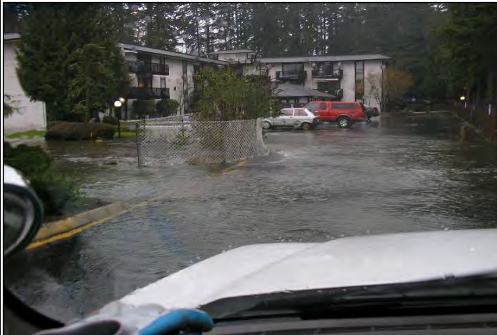
December 3, 2007 overtopping of existing Casa del Rey Culvert.
