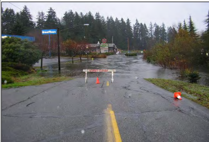
December 4, 2007, Flooding of Old 196th looking east
