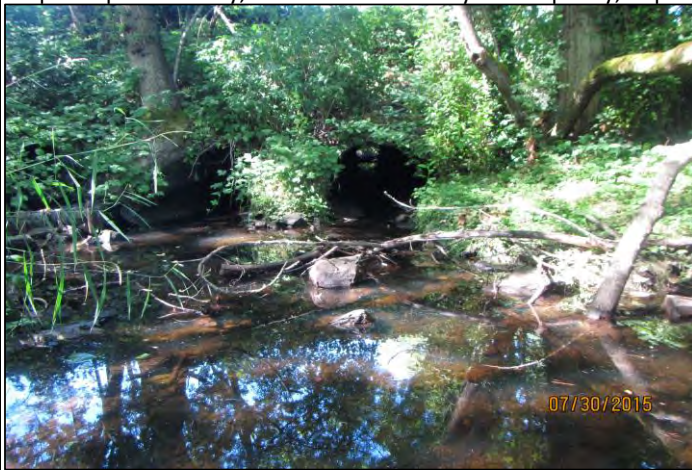
Looking upstream to outlet of existing 196th St SW culverts.
