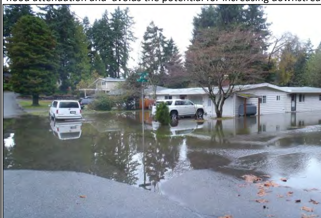
November 19, 2012 flooding of residential properties near 189th St SW.
