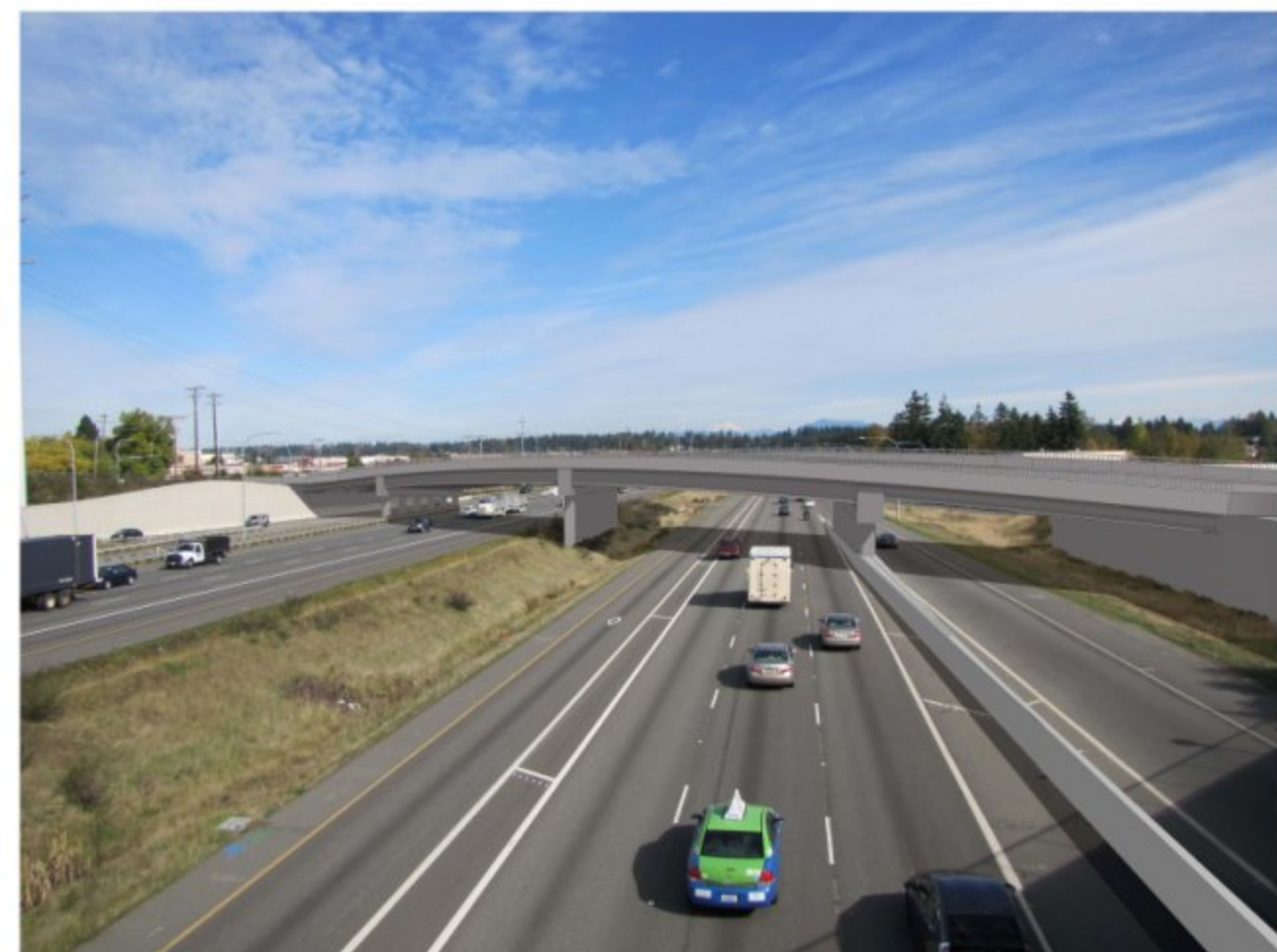
B I-5 LOOKING NORTH AT POPLAR WAY EXTENSION BRIDGE
